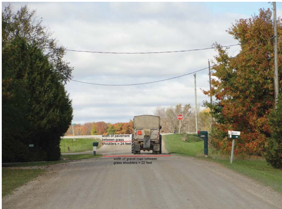
The width of the gravel surface between the grass shoulders measures 22 feet. The pavement width measures 24 feet.
