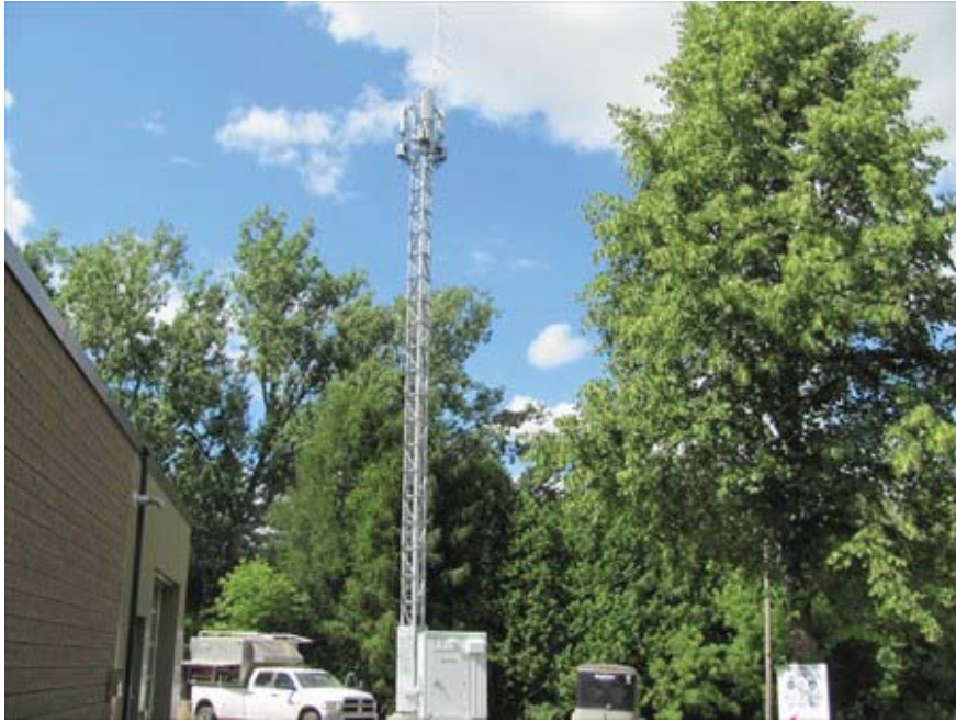
Bell Fire Hall replacement in Shelburne, ON.
