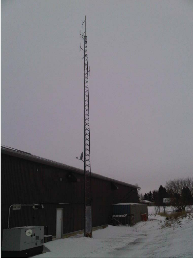
Dundalk, ON Fire Hall Original Tower
