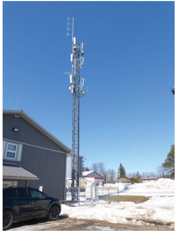
Dundalk, ON Fire Hall New Tower
