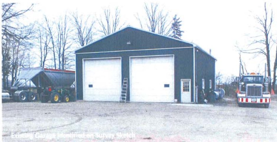
Existing Building Identified on Survey Sketch
