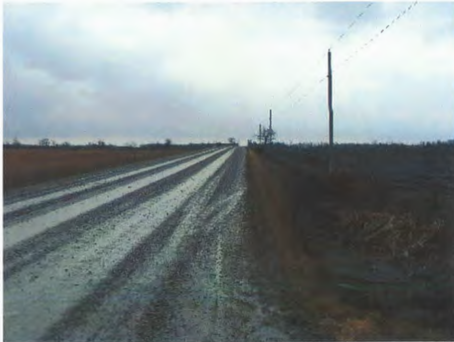
View to the South
