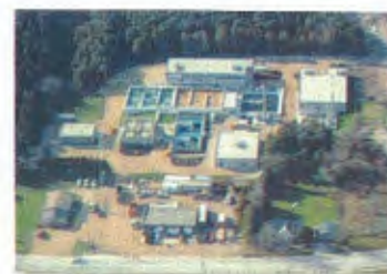
The new Elora wastewater treatment plant will improve river water quality for the world-class brown trout tailwater fishery
