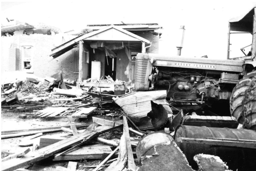
Photo of damage from the May 31, 1985 tornado. Photo from the Arthur and Area Historical Society.
